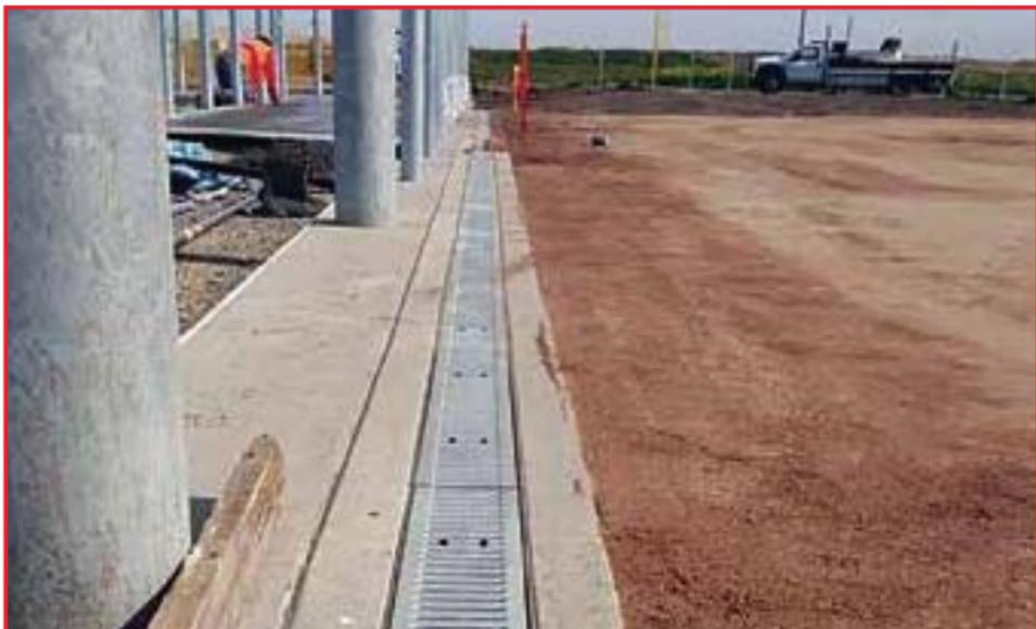
Hydrotec also met the specifications. Both Class A Grate and Class C Grates were specified; in the end, Class C Grates were installed throughout the site because they accommodate vehicular traffic. In order to ensure that the surface would withstand the weight of construction vehicles, and maintenance equipment in the future, Class C was deemed the more suitable choice.
