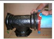
Step 2). Slide the mechnical joint gland and snap-on gasket combination onto the pipe spigot and insert the pipe-end and gland/gasket assembly in to the mechanical joint opening.
